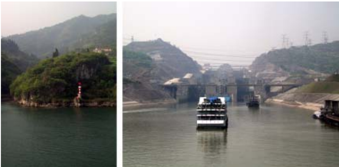
Figure 6: Navigation facilities in the Yangtze River. On the left, river beacon; on the right, the Three Gorges double-way five-step ship-lock (Credits: Kay Young).
