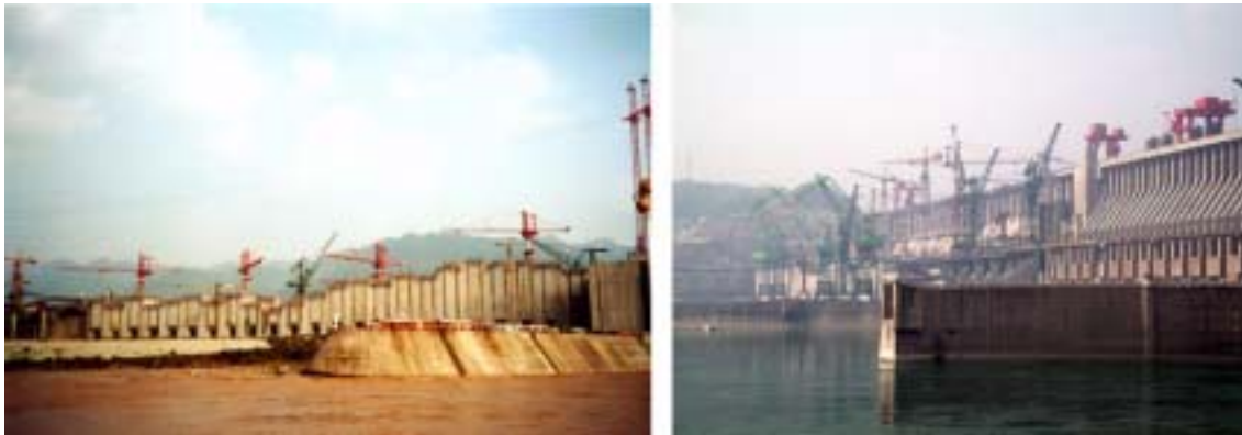
Figure 4: Images of the Three Gorges Dam construction. On the left, works on the left bank section of the dam, in September 2001 (Credit: Benjamin Lyons); on the right, works in the right bank dam, in April 2006 (Credit: Kay Young).
