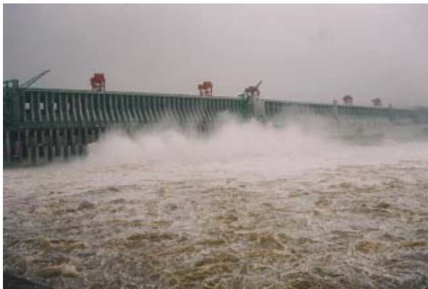
Figure 5: Three Gorges Dam sluice gates discharging water (Credit: Three Gorges Probe).
