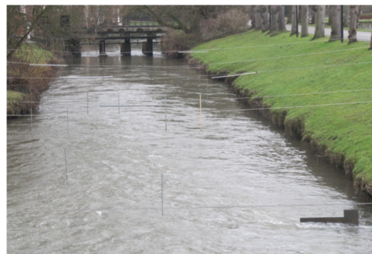
Gabions and one single groyne protect the bank
